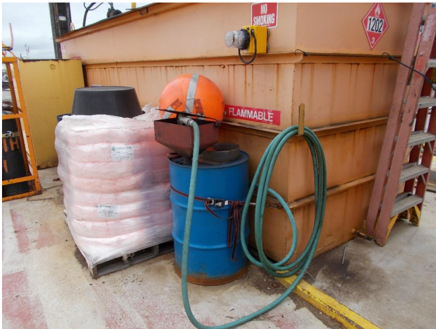
Figure 4: Drip pan for automatic shut-off nozzle and absorbent spill clean-up materials next to fuel tank.
